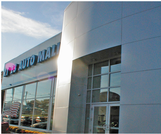
A view of the new exterior.
