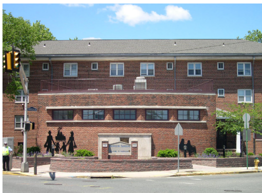
New landscaping beds, retaining walls, and silhouettes.
