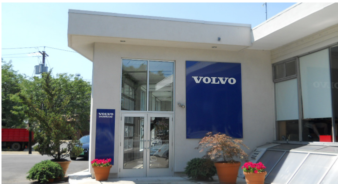
The new main entrance at the new showroom.
