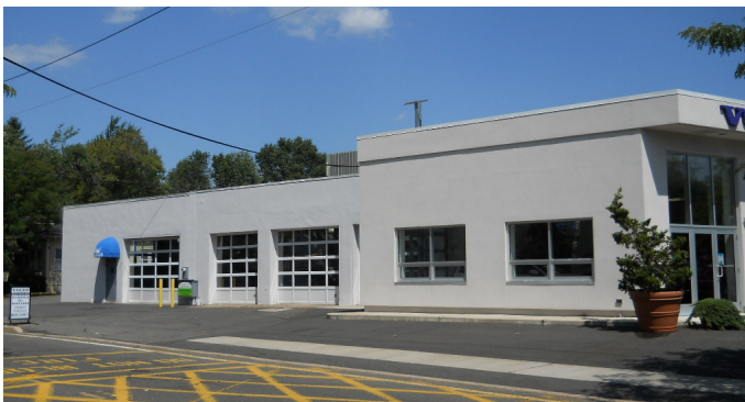
The side elevation showing the new showroom on the right and the new service bay on the far left.
