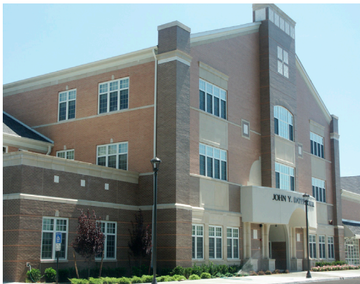
A view of the completed front exterior.
